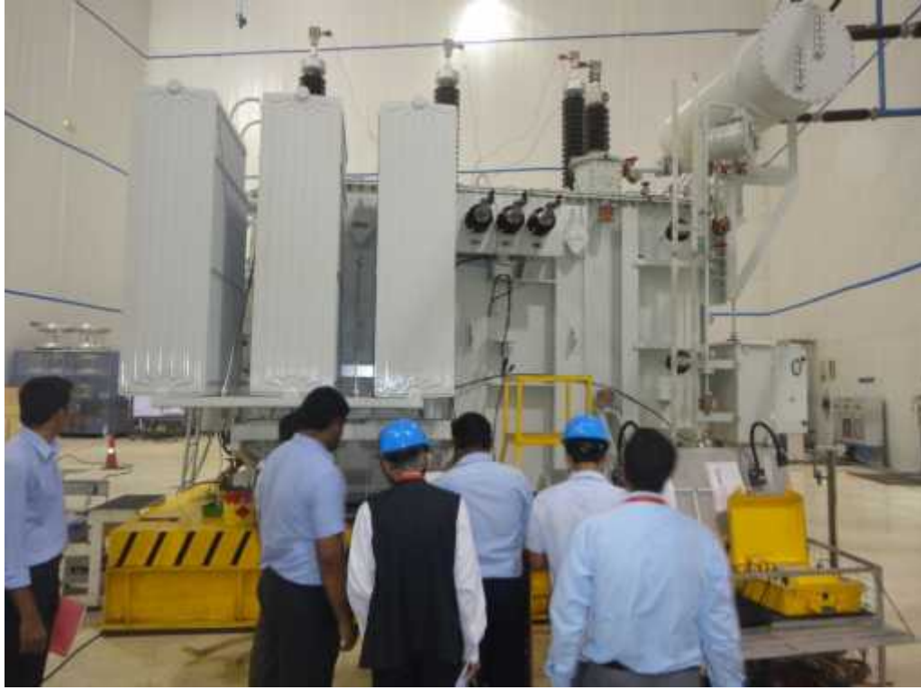
Inspection of Transformer
