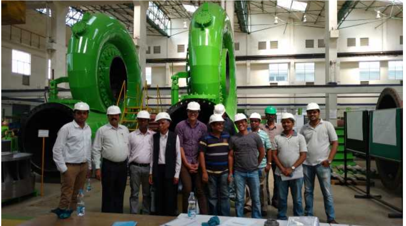
Inspection of Turbine
