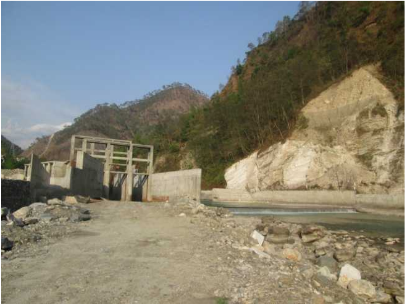
Headworks from downstream
