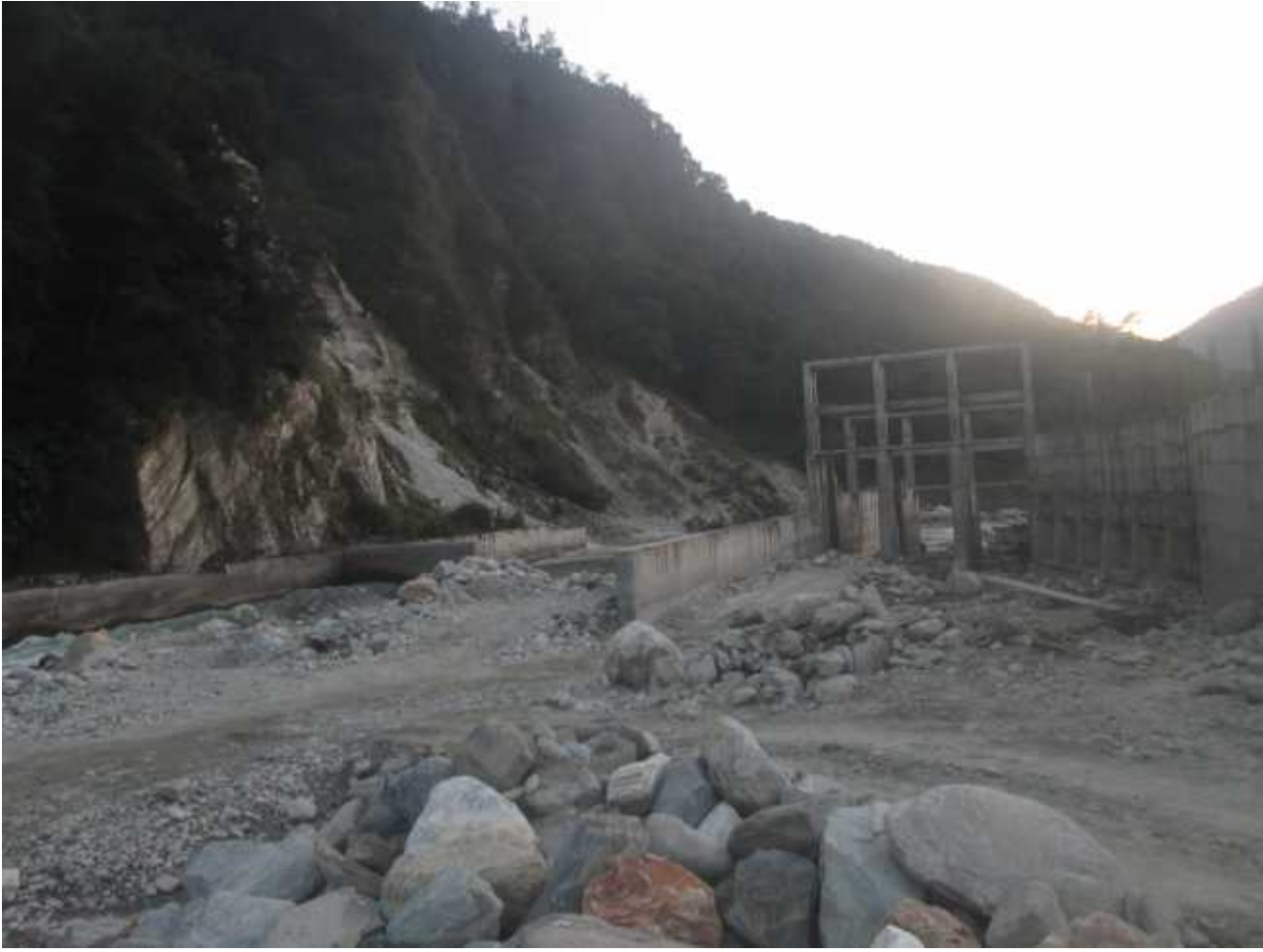
Headworks from upstream
