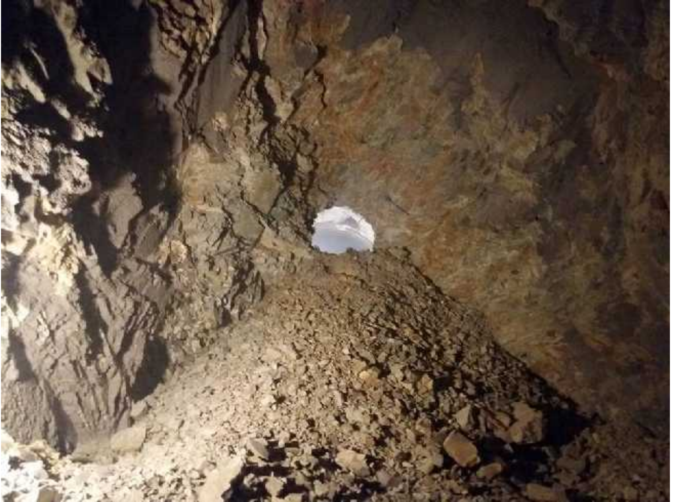
Breakthrough of 1326 m section between outlet and Adit-2
